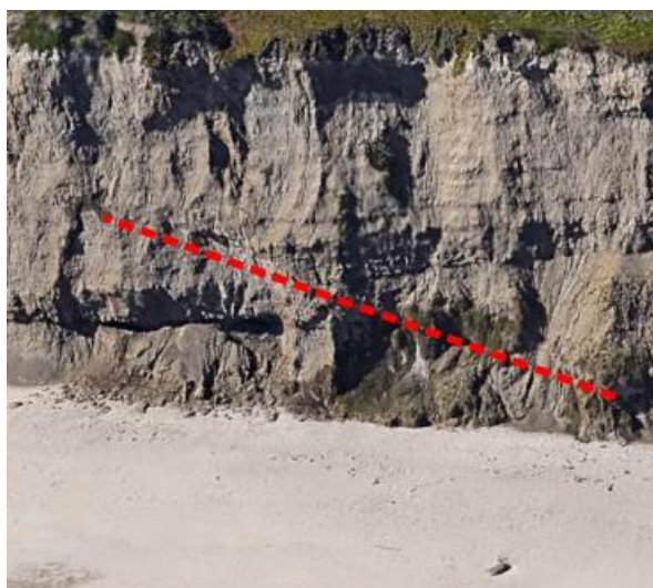
(Fig. 4a) a reverse fault seen in an outcrop of the bluff in the moss beach study area.
